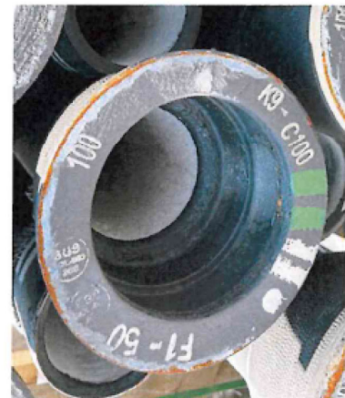
Ductile iron pipes with push in flexible joints (K9)
